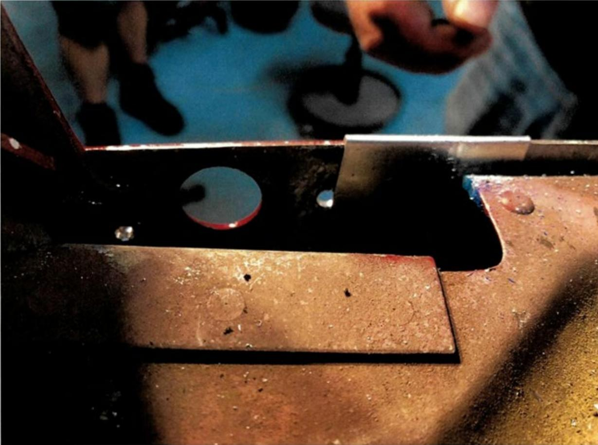
**Figure 13: After removing reinforcement angle cutoff**
