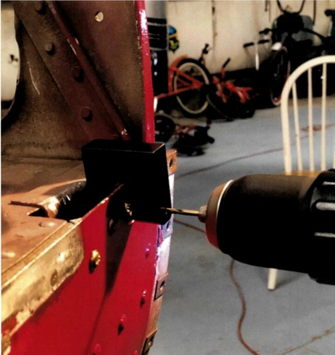
**Figure 31: Drill pilot hole through reinforcement splice**
