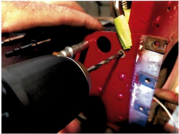
Figure 21: Drill aft tail cone reinforcement hole
